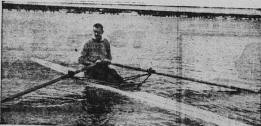
NEW TYPE —The Danish rowing club in Copenhagen has constructed a new type of single sculler, using Fibreglas instead of wood. Weighing about 30 pounds, the sculler was used by Jenson of the U. S. is trying out the new craft, the frame of which is light metal.
