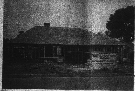
FRONT VIEW—Typical of the many small homes under construction in Anaheim today is this one at 555 So. Palm, designed by John Swint. A well constructed frame house, it will be finished in light green stucco combined with siding painted yellow, and a four foot facing of red brick at the front. The cedar shingle roof will be left natural.
