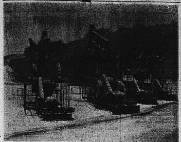
WELL PUMPS —This type of oil pump, low and less offensive than older types, will be utilized over all wells located on city lease. Only the portable derrick will be used in drilling. Tanks in background are carefully concealed.
