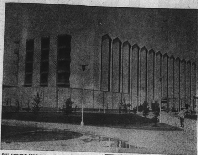
GETS FINISHING TOUCHES — Orange State College's great new Science Building is in the final stages of completion and being made ready for the fall semester. Scene from its roof-top are other parts of current $20 million project. (Gazette Photo)
